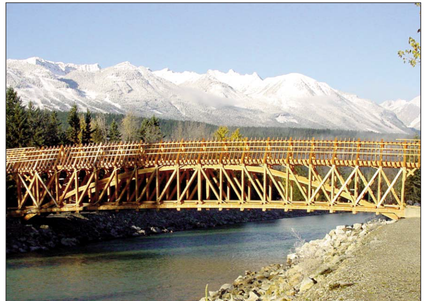
Kicking Horse River Bridge, Golden, B.C. – built as a Timber Framers Guild project. West Forest Timber Inc. supplied the curved timbers sawn from naturally curved logs so the grain follows the arch providing great strength.
